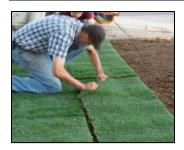
Keep the rolls snug against each other without overlapping. A sharp knife makes clean cuts for a perfect fit. Avoid leaving small strips at outer edges as they will not retain moisture. On slopes, place the turf pieces across the slope rather than down. After you've laid about 200-300 sf of sod, spray it with a light mist from your garden hose. This will prevent the sod from drying out before you are finished with your complete project.
