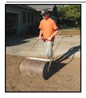
Roll the area lightly with a lawn roller (available for rent at local hardware store) 1/3 full of water. This will firm the soil surface and reveal low areas that may need additional soil. Apply lime, if needed. We recommend an application of dolomite or agricultural grade limestone at the rate of 50 lbs per 500 square feet. Rake area lightly. Final grade should be one inch below the sidewalk/driveway. Water the area lightly to provide a moist base for the turf.
